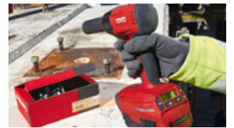
HST3 setting with SIW-6AT impact wrench
