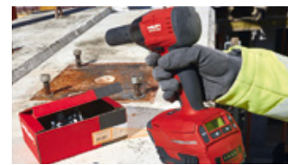
HST3 setting with SIW-6AT impact wrench
