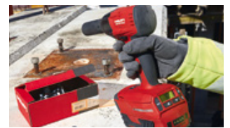
HST3 setting with SIW-6AT impact wrench
