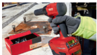
HST3 setting with SIW-6AT impact wrench
