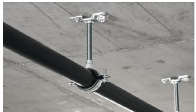
In many cases, mechanical fasteners that require a hole to be drilled (and dust emitted) are simply over-designed for the loads they have to carry. Direct fastening tools can often yield a fixing point that is fit for purpose. It's quick to make the fastening point and it doesn't generate any dust.
