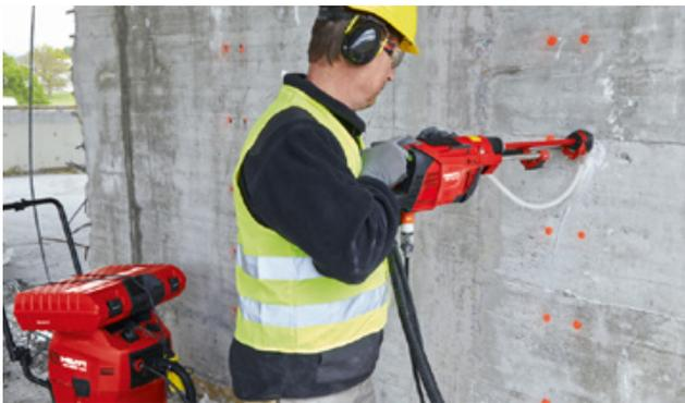
Holes for anchors or rebar can be cored instead of hammer drilled. Slurry can be collected with a water recycling unit, so slurry isn't spilled only to turn into dust when it dries. Penetrations can be cored instead of broken out with a combination of cutting and breaking, which also reduces dust emission.
