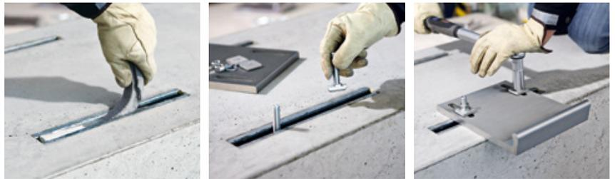
Instead of post-installing anchors with the resulting dust emission from the hole, it is possible to cast-in an anchor point prior using a channel. T-bolts can be slotted into to create a fixing point
