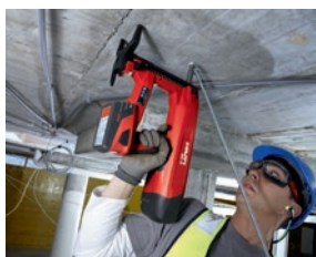
Threaded rod attachments to concrete
