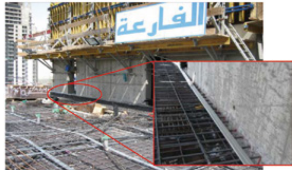
Slab connections
