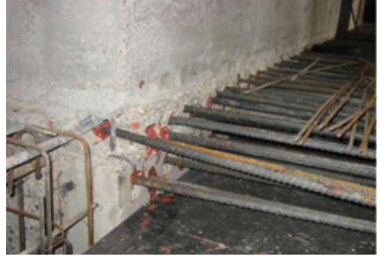
New slab constructions
