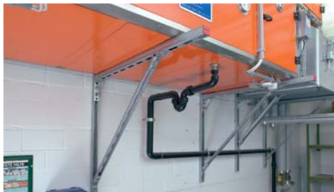
Reliable assembly of demanding air conditioning systems.
